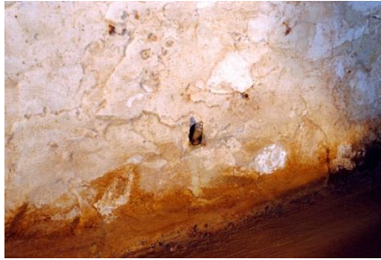
Packer is set in place
