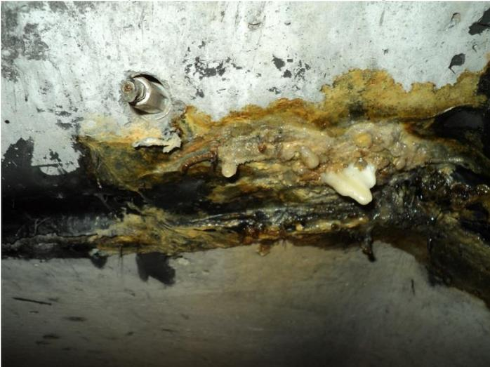
This shows the proper depth to set the packer and also the discoloration & deterioration of the leaking tunnel.
