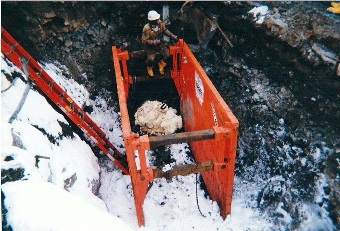
The expansiveness of HyperFlex, coupled with its adhesion and flexibility, make it an ideal medium for filling voids, in this case a 48" pipe at an inactive steel mill.
