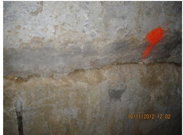
These photographs show the dry basement wall after our grouting project. The darker areas are from the hydraulic cement we used to repair our injections sites.
