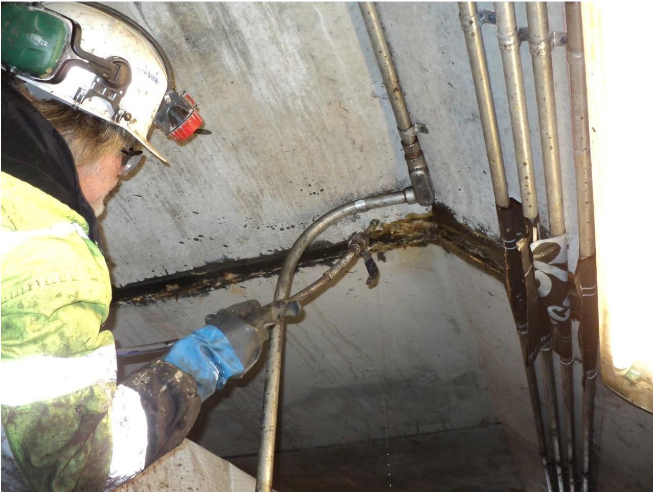
This shows our Sr. project Manager injecting HyperFlex into the joint.
