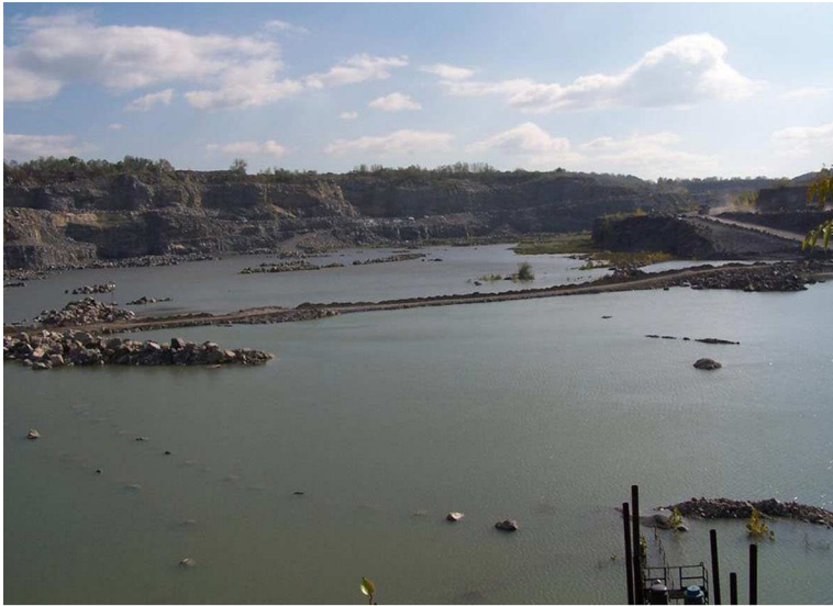
Quarry Karst Leak, N.Y. 30,000 GPM
