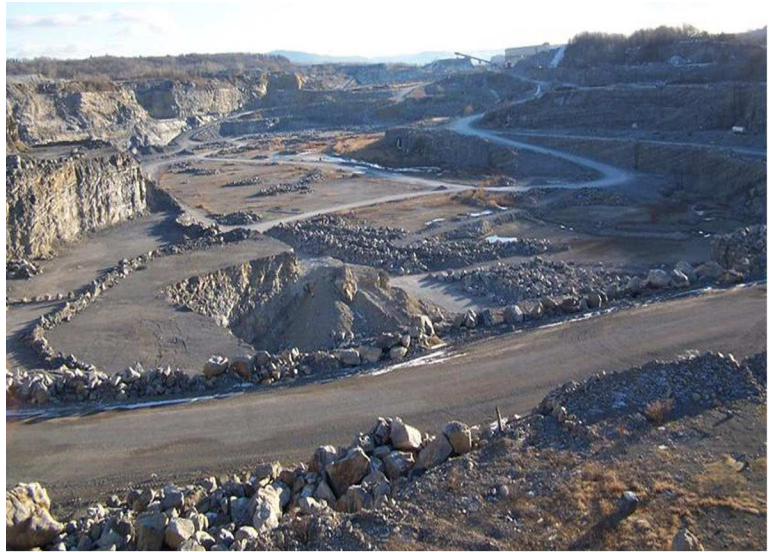
Quarry Karst Leak N.Y. 0 GPM
