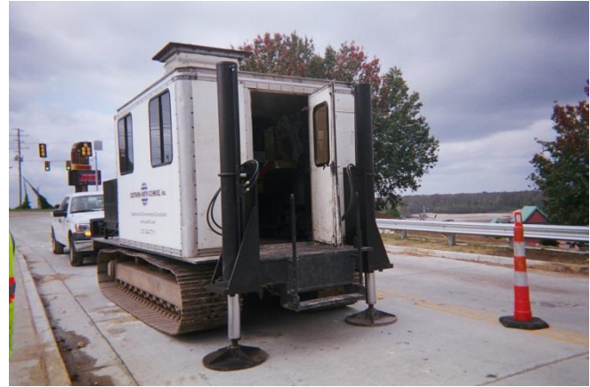
Compaction Penetrometer used to measure ground compaction after grouting.
