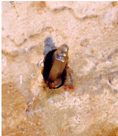
This shows the correct way to set a packer for injection
