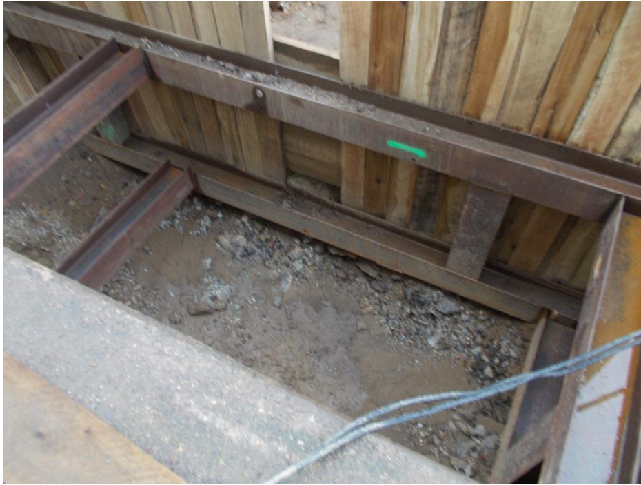
The excavated pit at the conclusion of our project
